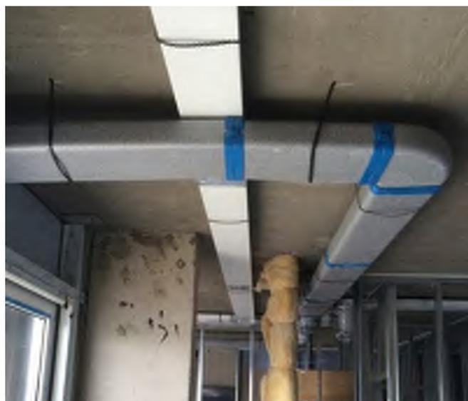
*Ducting at Site 2 – Rigid duct installation. Straight duct runs using proprietary bends where needed. Intake/exhaust ductwork is pre-insulated (grey ducting). Ducting mechanically connected and fastened throughout*
