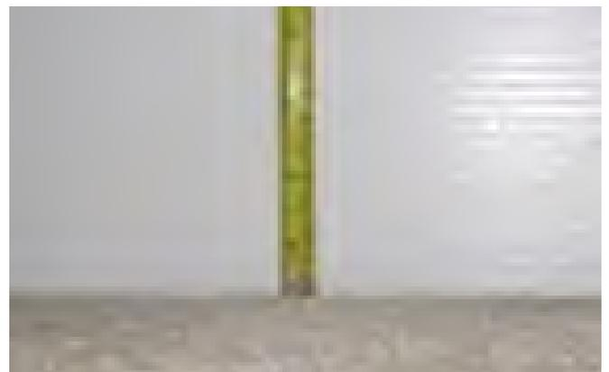
Site 1 – Example of inadequate door undercut
