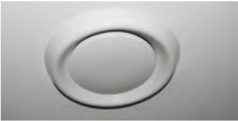
Site 2 – Example of room extract air terminal with inadequate air gap setting, leading to higher flow resistance and localised air velocity noise
