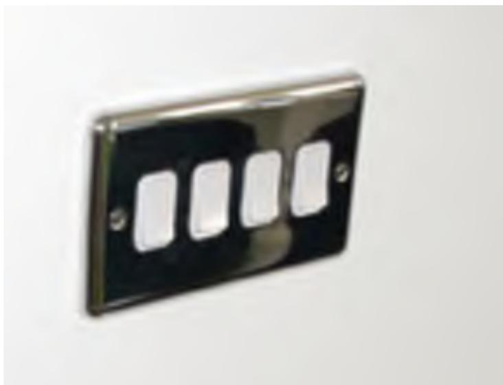
*Site 4 – Example of multi-gang switch. One of these is to boost the fan, but there is no labelling to tell the user which one*
