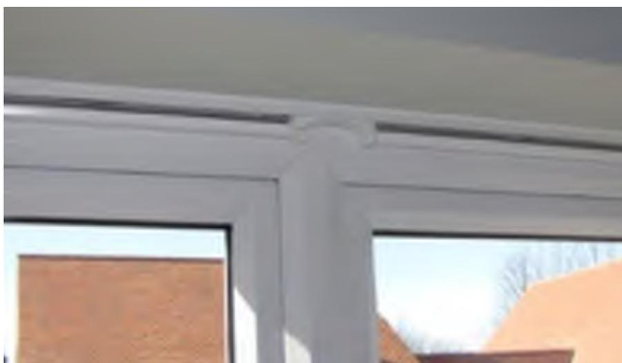
**Trickle Vents at Site 1 – Over-provision of trickle vents at Site 1. Two ventilators fitted with approximate EQA of 5800mm<sup>2</sup>. One trickle vent with EQA of 2500 mm<sup>2</sup> would meet ADF guidance.**
