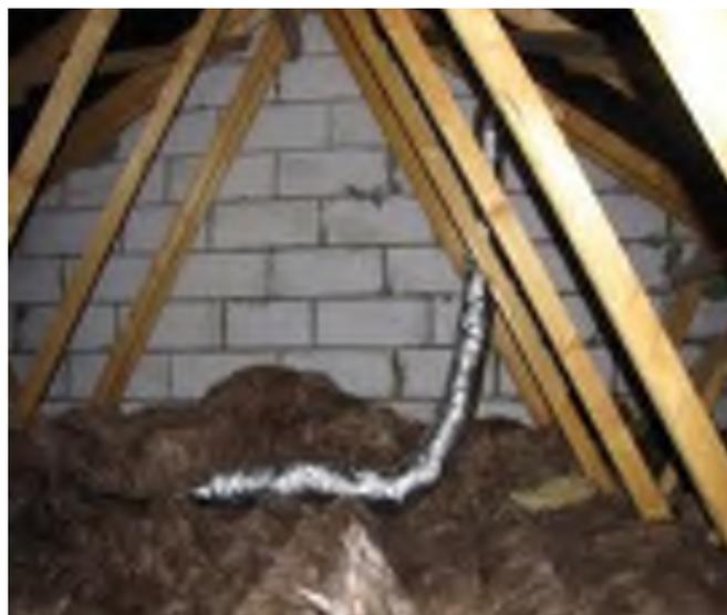
*Ducting at Site 3 – Long looping ducting could cause condensation to build up and increase the required fan power*
